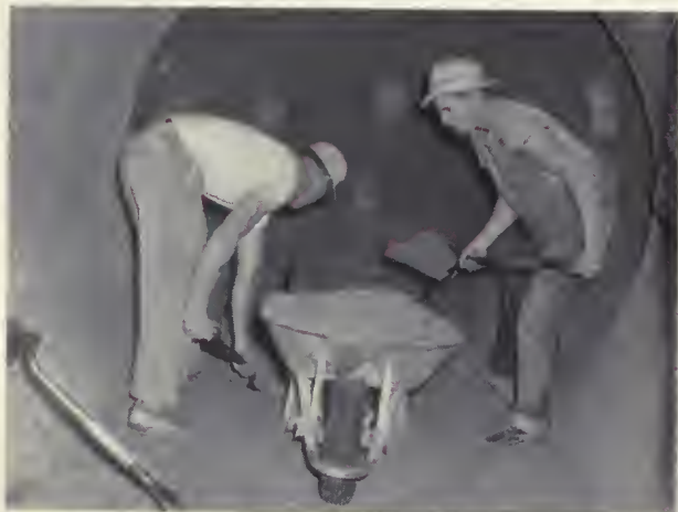
CLEANING UP the inside of a siphon under Highway 80 (top photo). At lower left, Pumping Plant No. 1 as it began to take shape last July. At lower right, on the same day, men were working on the discharge tubes for Pumping Plant No. 2.
